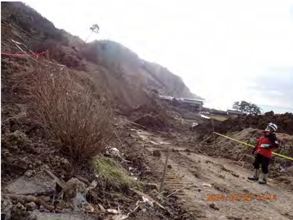
仁江町の地すべり地内の状況(2月3日)。図21の横軸80m付近の道路まで掘削を進めた状況。切り立ってしまい、これより上方の掘削が難しい状況になった。本文9ページ参照。 Situation of the landslide in Nie-machi (3rd Feb.). Deposit had been cut for searching from toe to about 80m of Fig.21, and the slope became too steep to progress. See also page 9.
